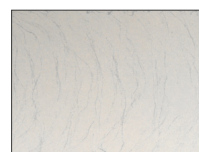
COVERAGE TOO LIGHT
